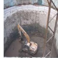
**11. The final foundation level at the base of the excavation will be cleaned and mapped in addition to the walls of the final lift. If any anomalous issues are discovered, additional geotechnical investigations will be performed in accordance with RG 1.132.**
