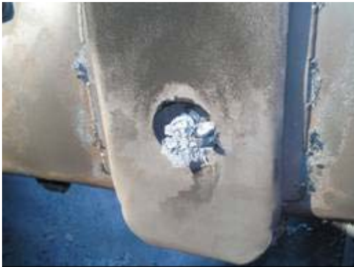
Figure 2-85 - Vent at stiffener
