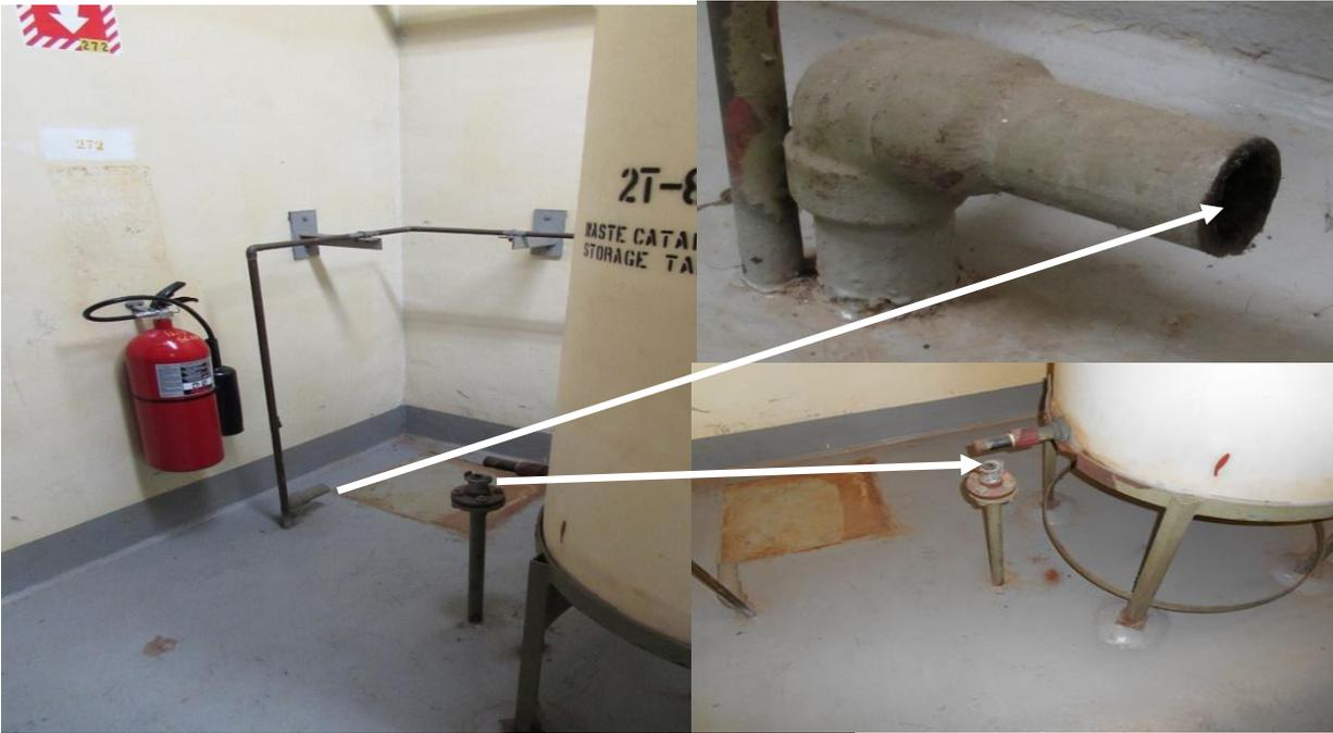
Above, pipes in the “as-found” images were cut and abandoned in place. They provided a potential pathway for flood water to flow into a flood-protected space underneath this room.
