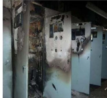
Non-fixed Magnet Blast Breaker (MBB), hung up by buses in the cabinet, was damaged during seismic strong motion
