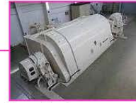
Short-circuit generator 15kV 2,500MVA 50/60Hz
