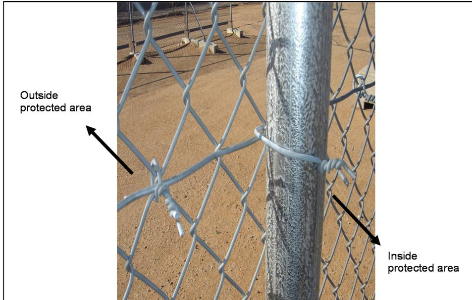
**Figure 33 Example of security fence wire ties**
