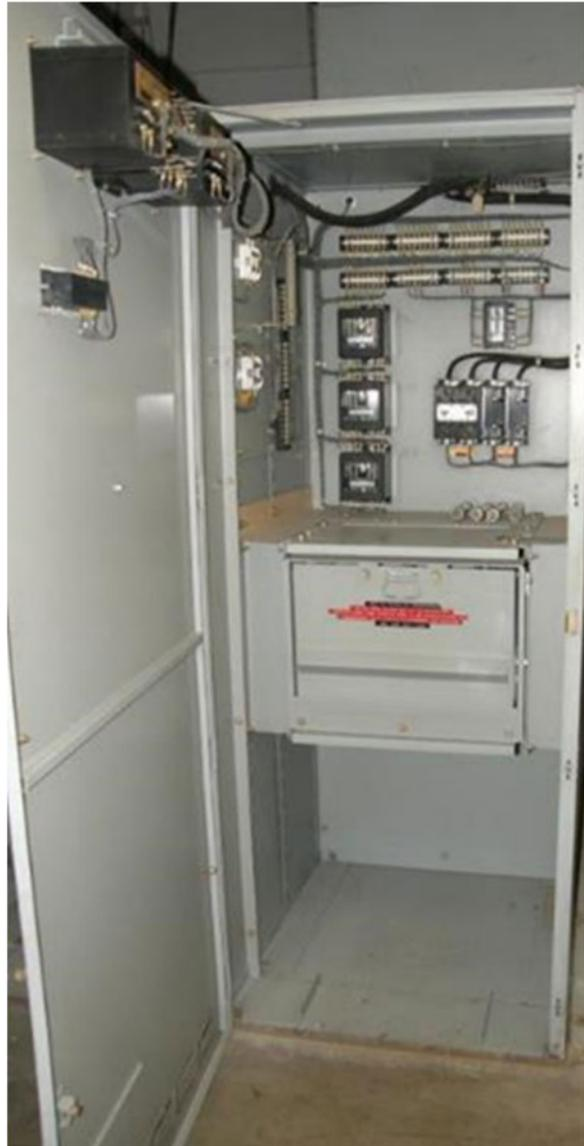
Figure 2-4. Photographs of the internal wiring of medium voltage switchgear.
