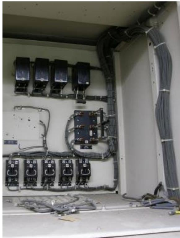
Figure 2-5. Photographs of the internal wiring from typical motor control centers.
