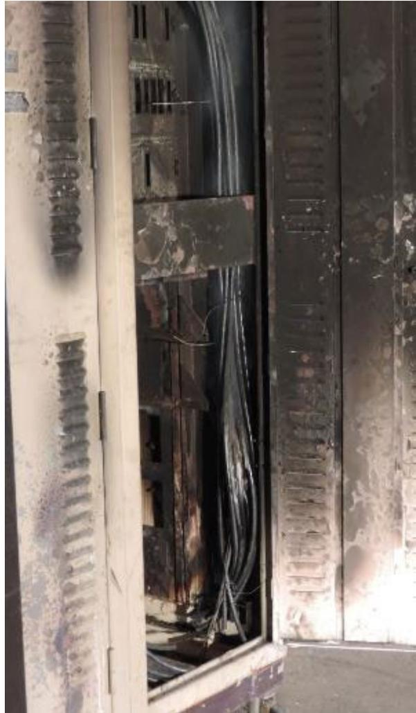
A close-up photograph of the cable bundles inside the enclosure. The cables are bundled together and appear to be in a compartment. The surrounding metal structure is dark and shows signs of heat exposure. |
