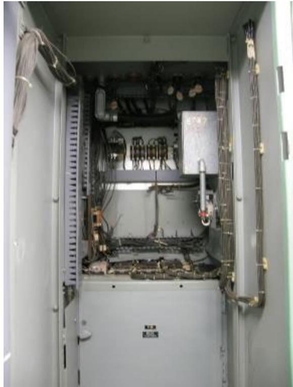
Figure 2-3. Photographs of the internal wiring of typical switchgear enclosures.
