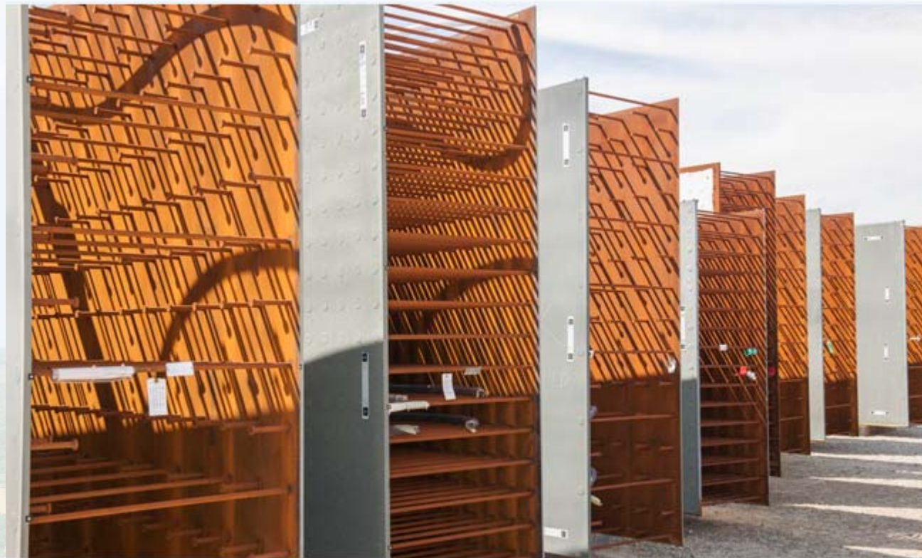
Vogtle Unit 3 shield building wall panels.
