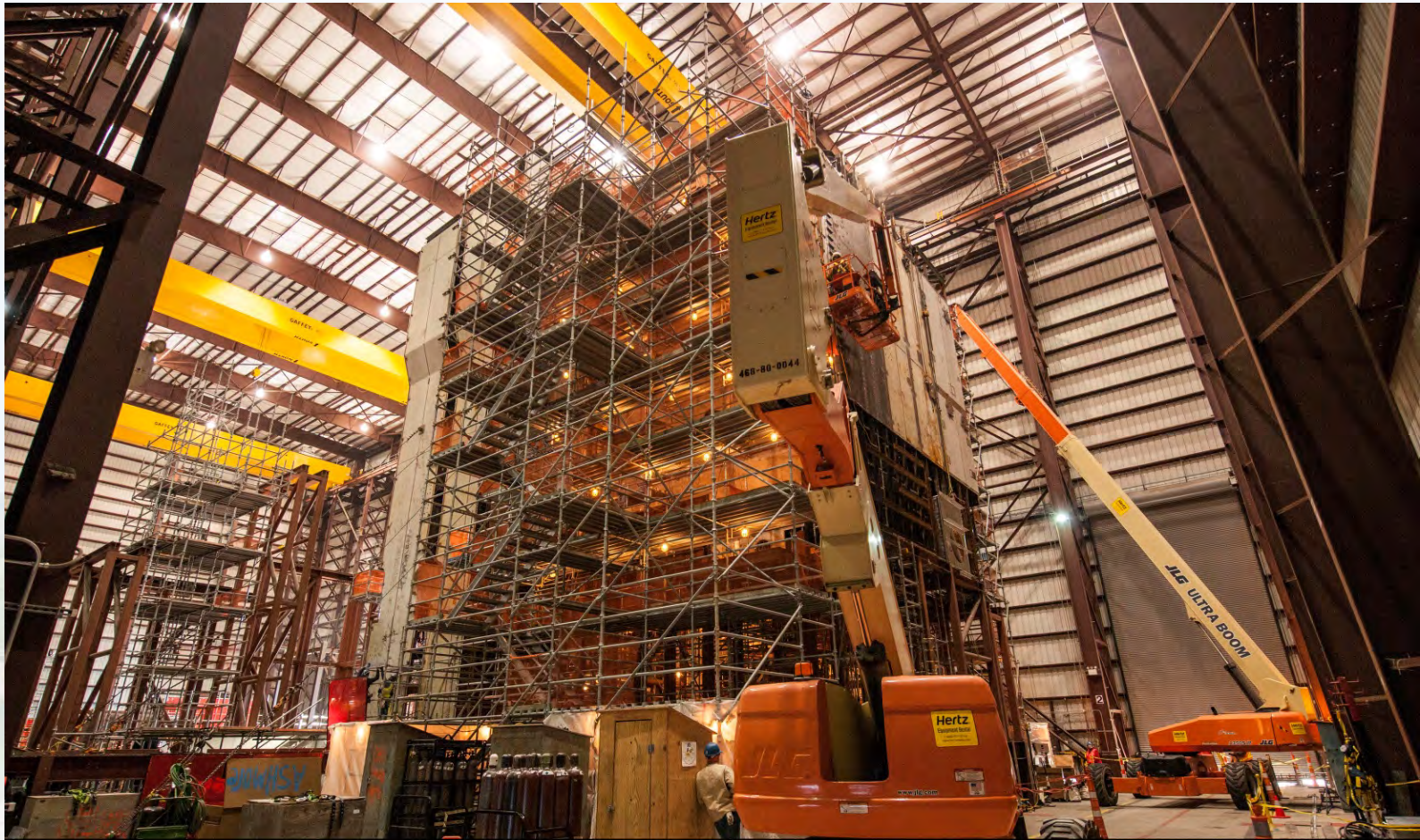
Vogtle Unit 3 CA01 module inside Module Assembly Building.
