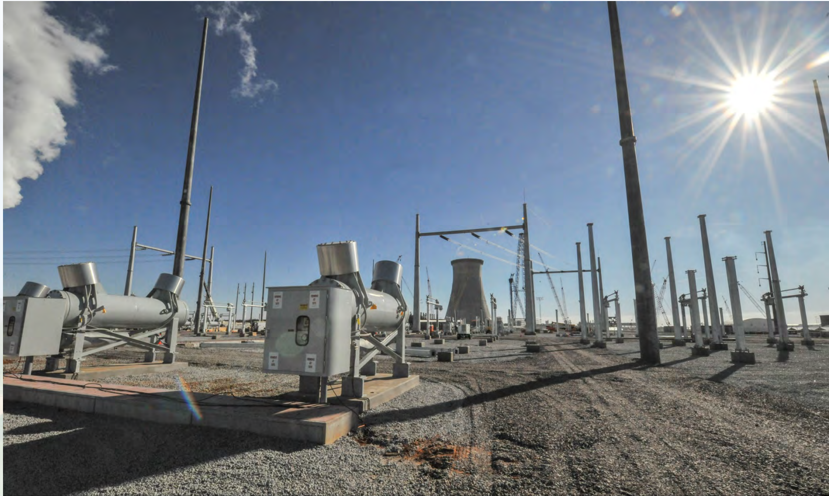
Vogtle Unit 4 500-kV transmission switchyard.
