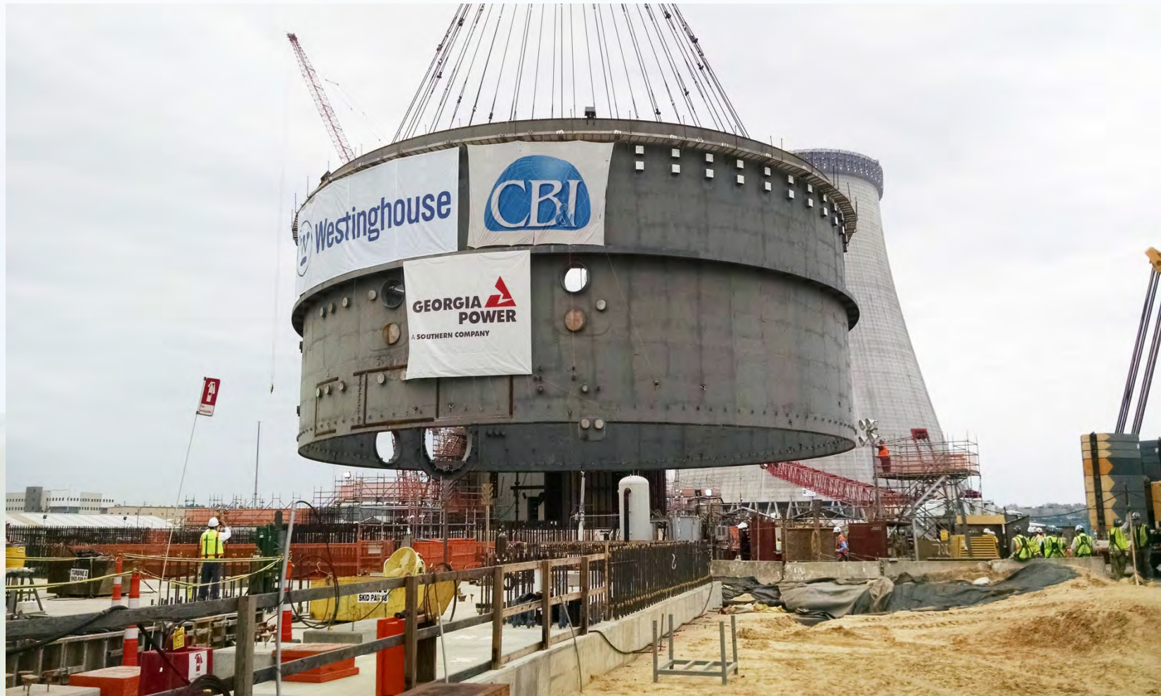
Vogtle Unit 3 lower ring placement
