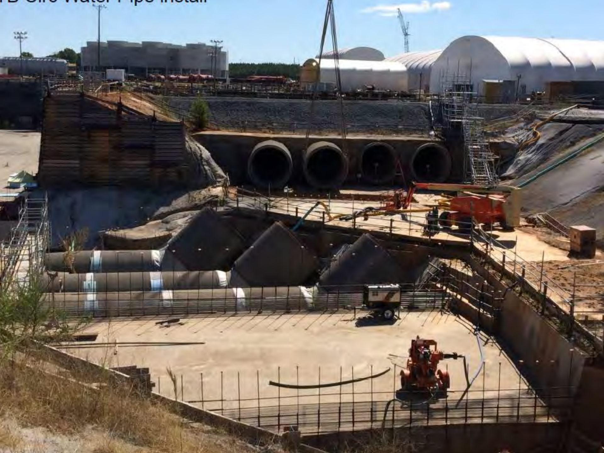
Drill Water Pipe Install
