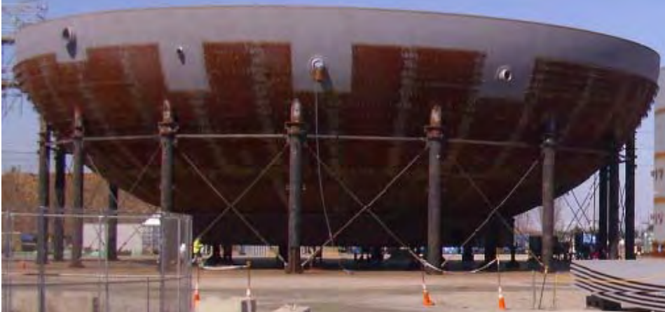
U3 Containment Vessel Bottom Head
