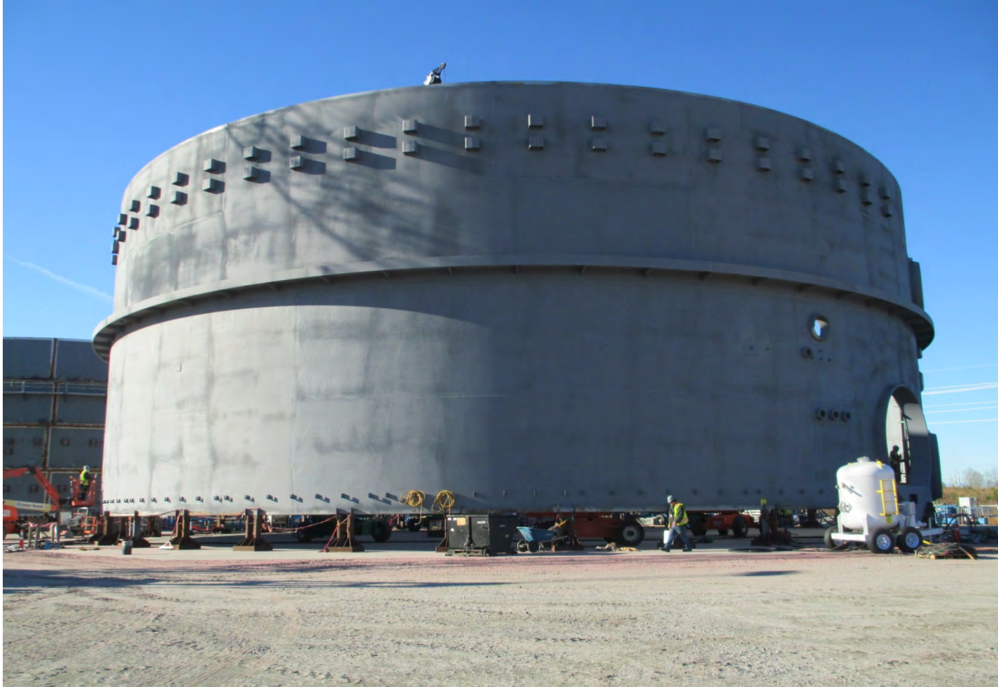
VCS Unit 2 Containment Vessel Ring 1
