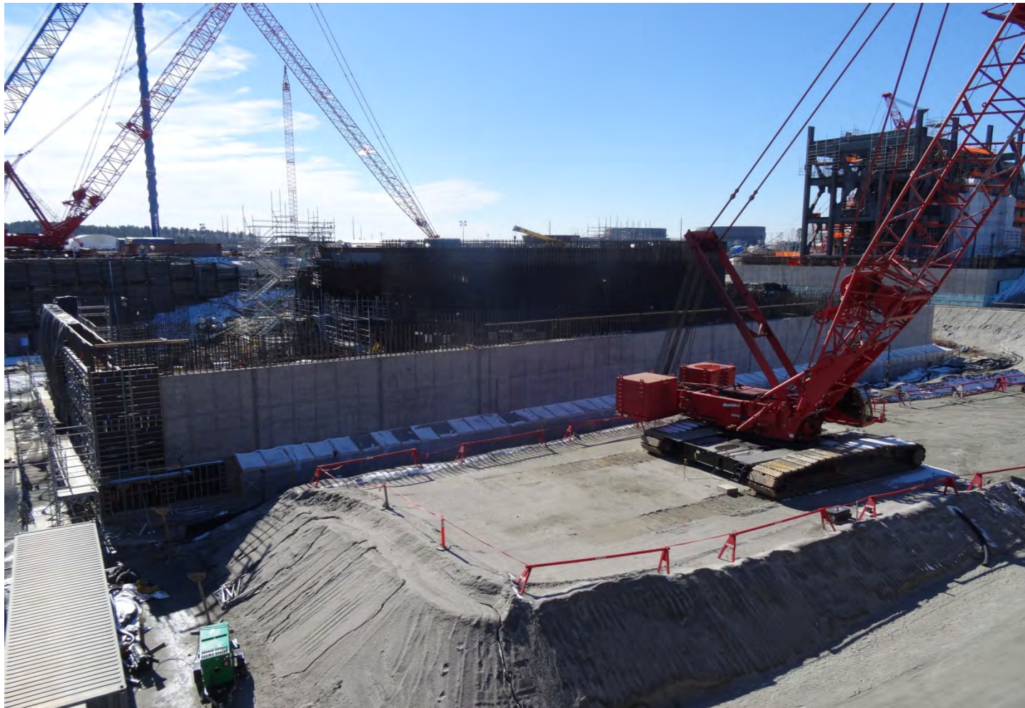
VCS Unit 2 Auxiliary Building Wall Construction
