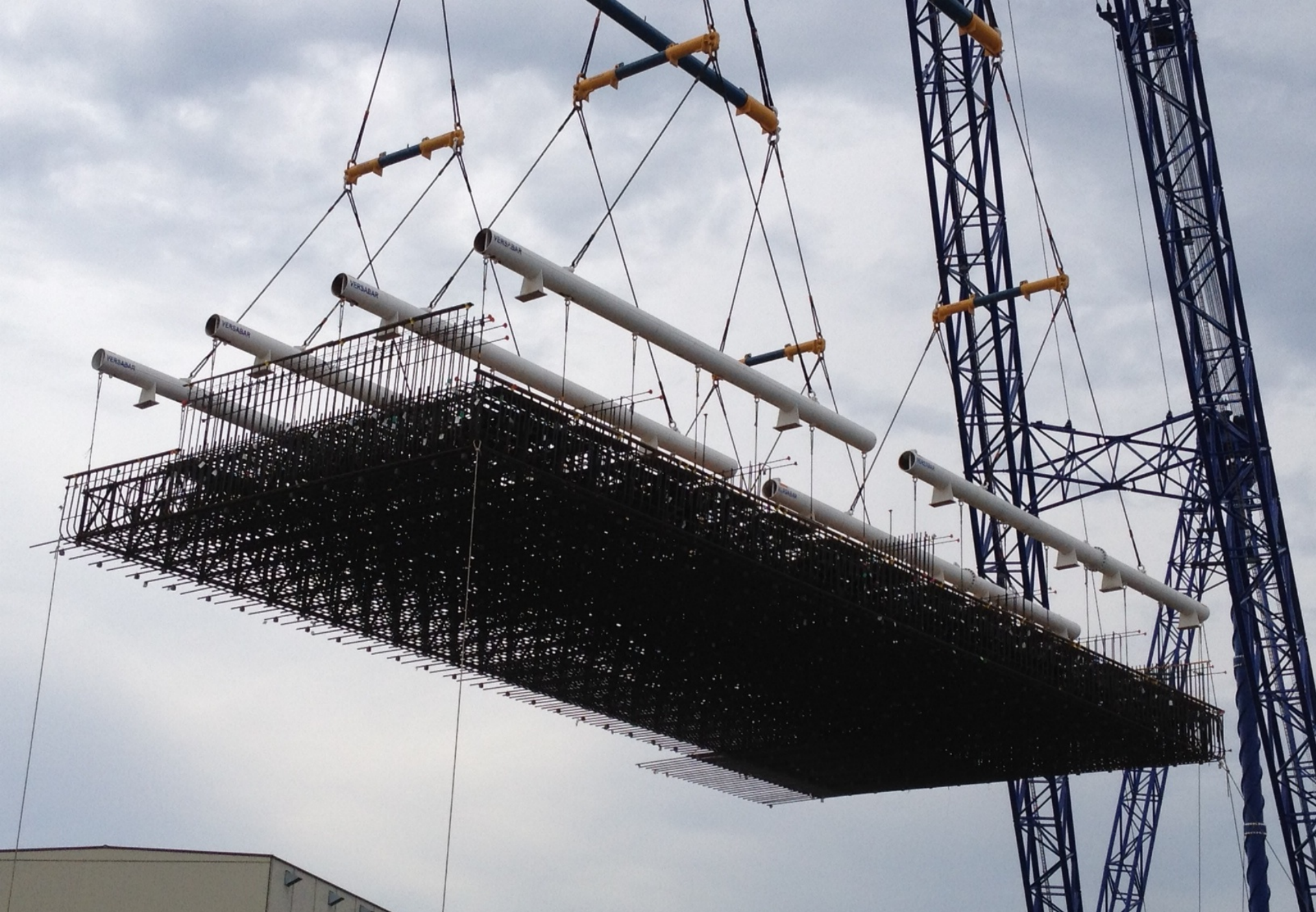
Unit 2 Nuclear Island Basemat Rebar Preassembly
