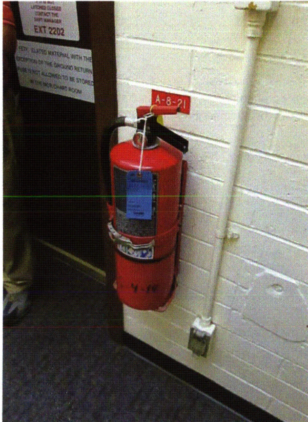
2PM06J - FIRE EXTINGUISHER SIEMIC MOUNTING Byron 1 & 2 005
