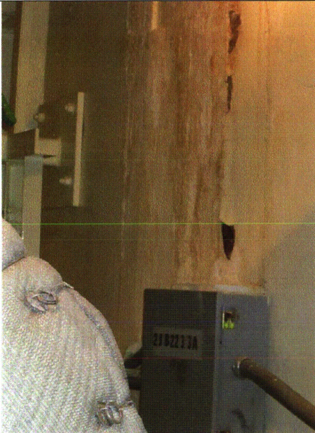
2RH01PA (WALL WATER LEAK) Byron 1 & 2 8-21-12 051
