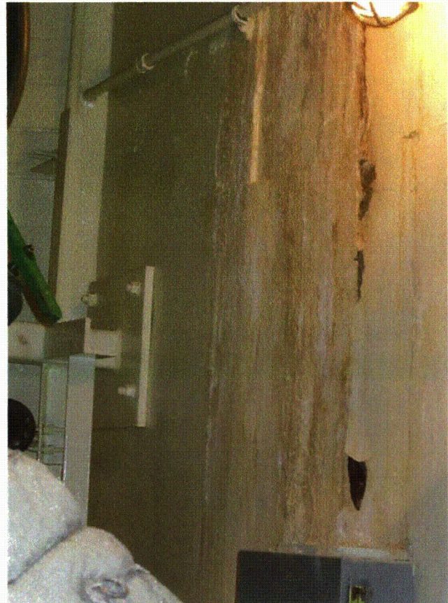
2RH01PA (WALL WATER LEAK) Byron 1 & 2 8-21-12 050
