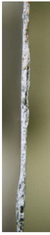
Boral edge showing oxidation and delamination EPRI TR-1013721
