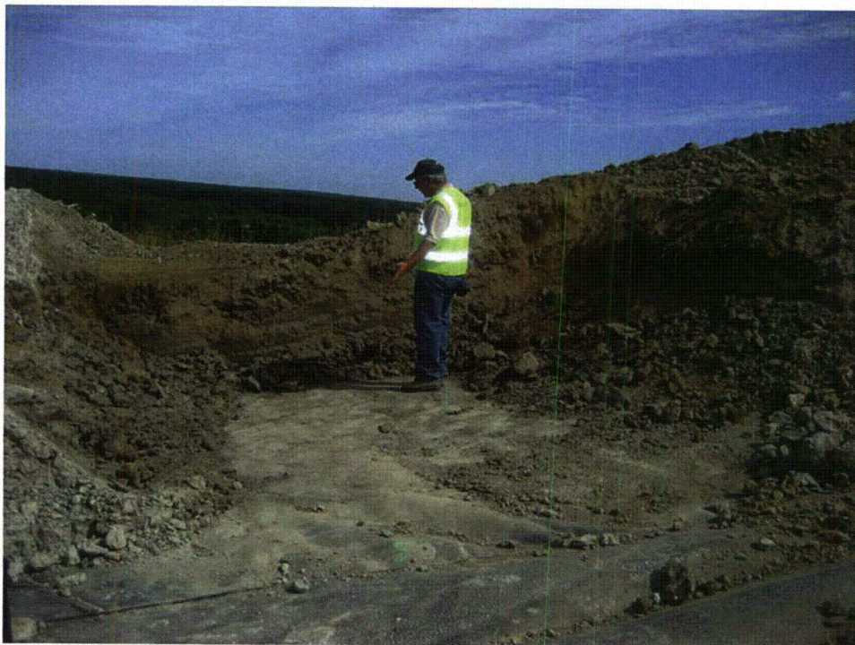
Fig. M. 20. Test Pit 2 after removal of overlying soil layer.
