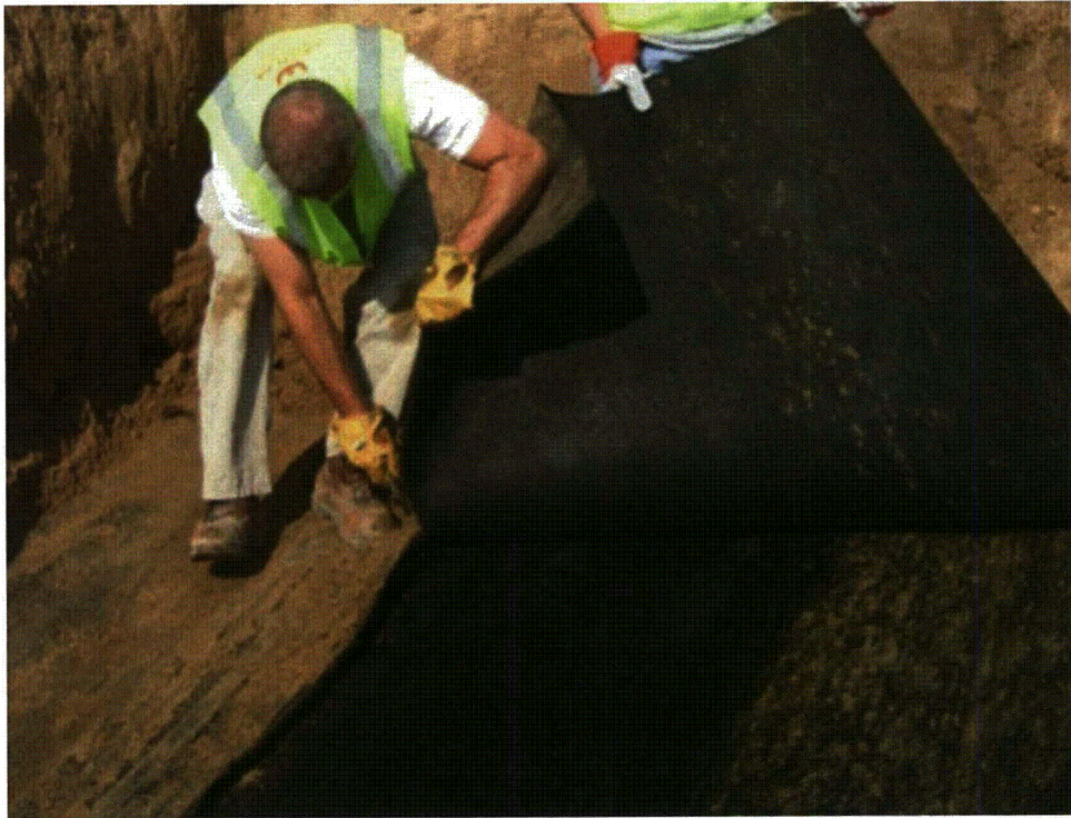
Fig. M. 10. Removal of GDL exposing GM.
