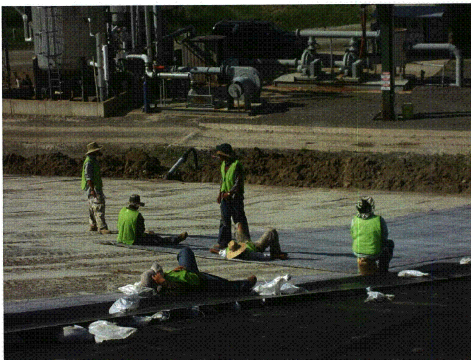
Fig. M. 28. GCL instillation team between rolls.
