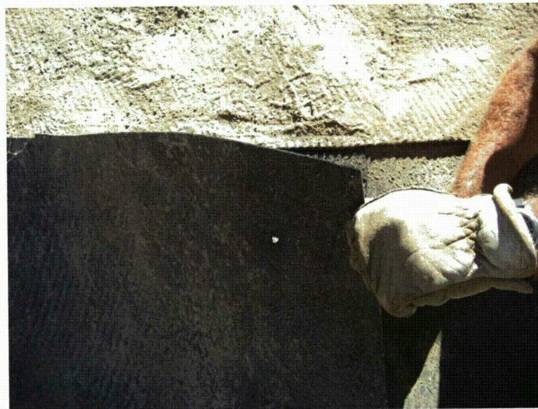
Fig A.6. Constructed defect in GM.
