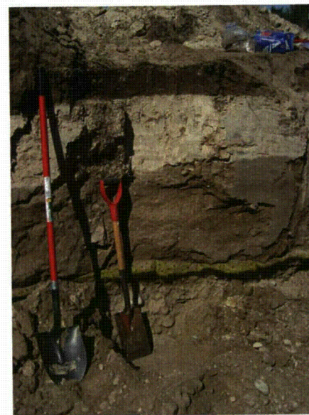
Fig. A.33. Alternative (ET) cover profile, veg. barrier visible.
