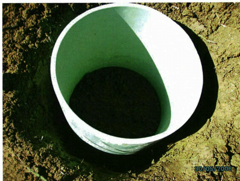
Fig. A.43. Installing TSB, rough bottom to avoid smearing.
