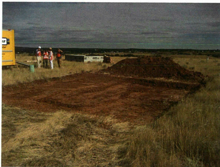
Fig. A.78. Vegetation layer removed for SDRI installation.
