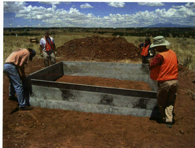
Fig. A.85. Setting SDRI in trenches.
