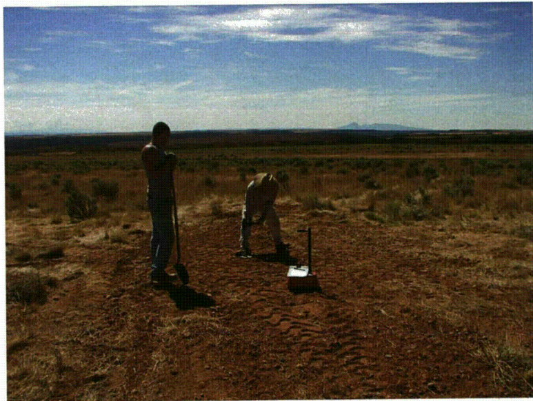
Fig. A.98. Ensuring re-compaction to initial dry density.
