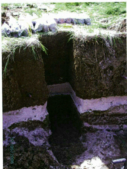
Fig. A.61. AO2 (capillary barrier) cover profile.
