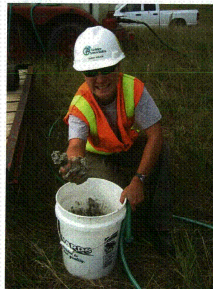
Fig. A.69. Mixing bentonite grout for TSB installation.
