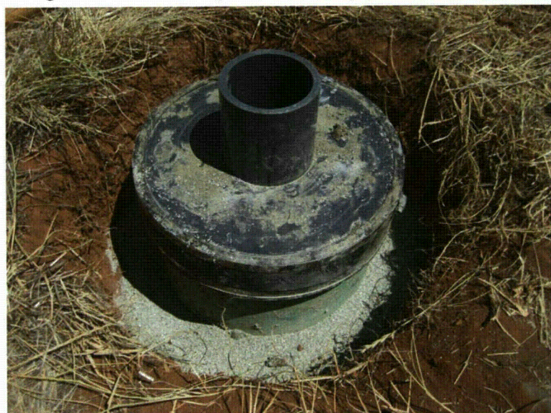
Fig. A.82. Sealing upper TSB section with granular bentonite.
