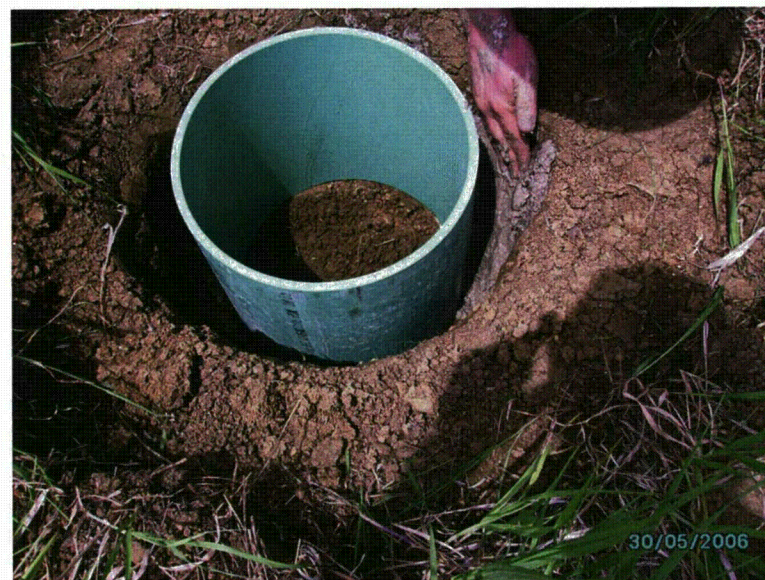
Fig. A.44. Grouting TSB with bentonite paste.
