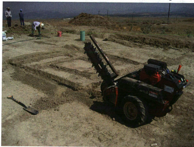
Fig. A.12. Cutting trenches for SDRI installation.
