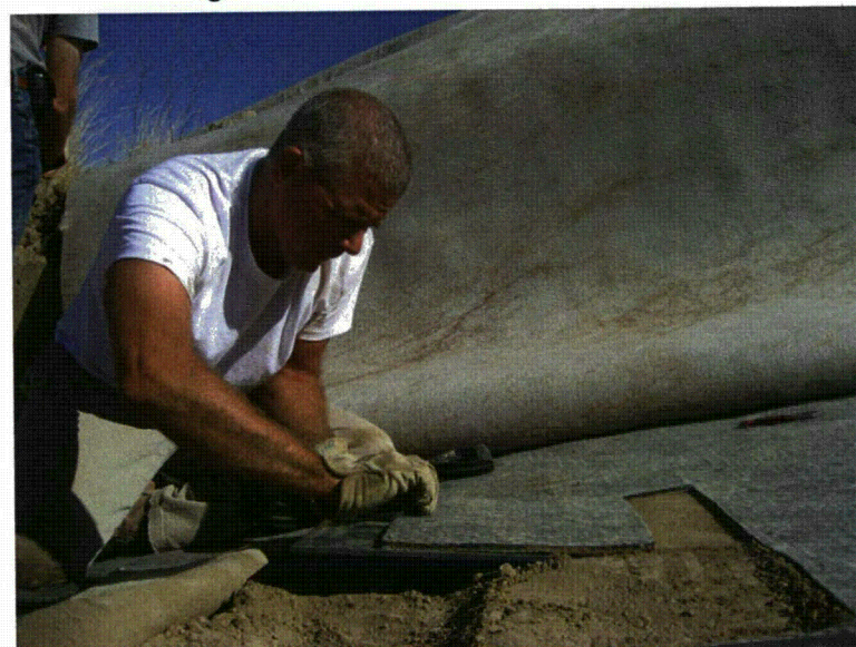
Fig A.8. Delicately plating GCL to avoid disturbance.
