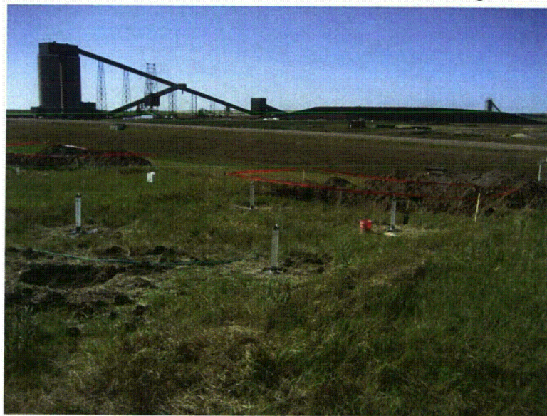
Fig. A.68. TSBs in operation, and test pits.
