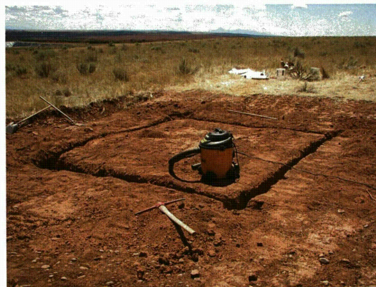
Fig. A.81. Cleaning site for SDRI installation.
