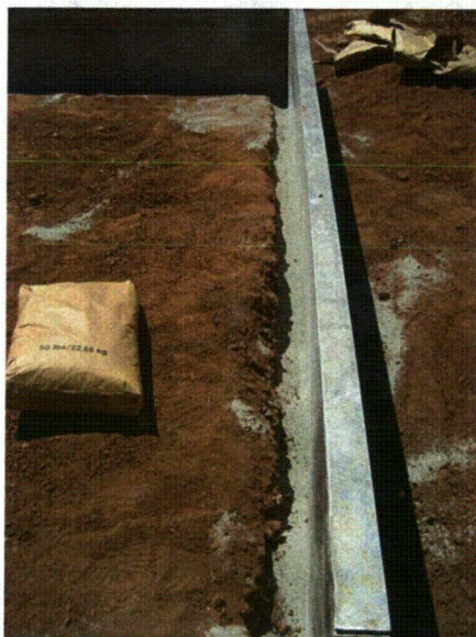
Fig. A.86. Sealing SDRI perimeter with granular bentonite.
