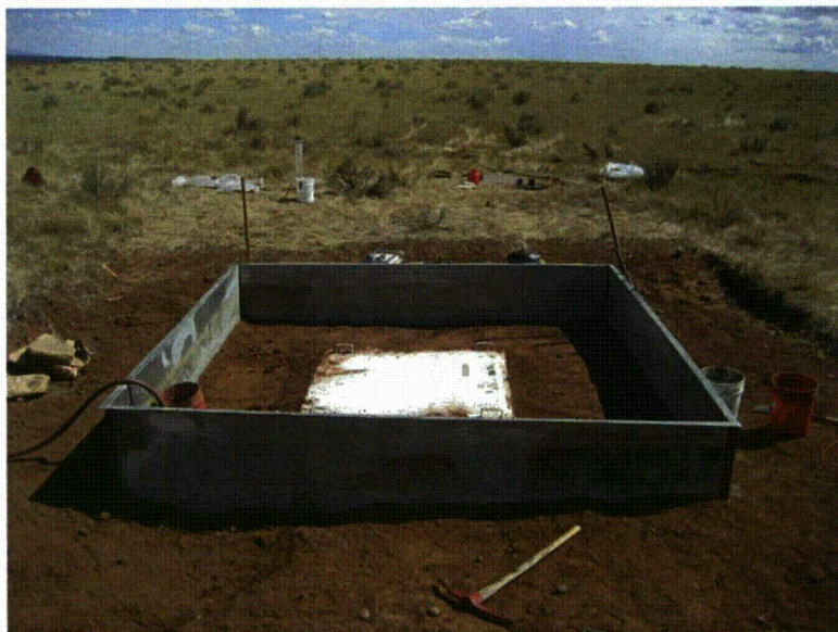
Fig. A.88. Installed TSB prior to operation.
