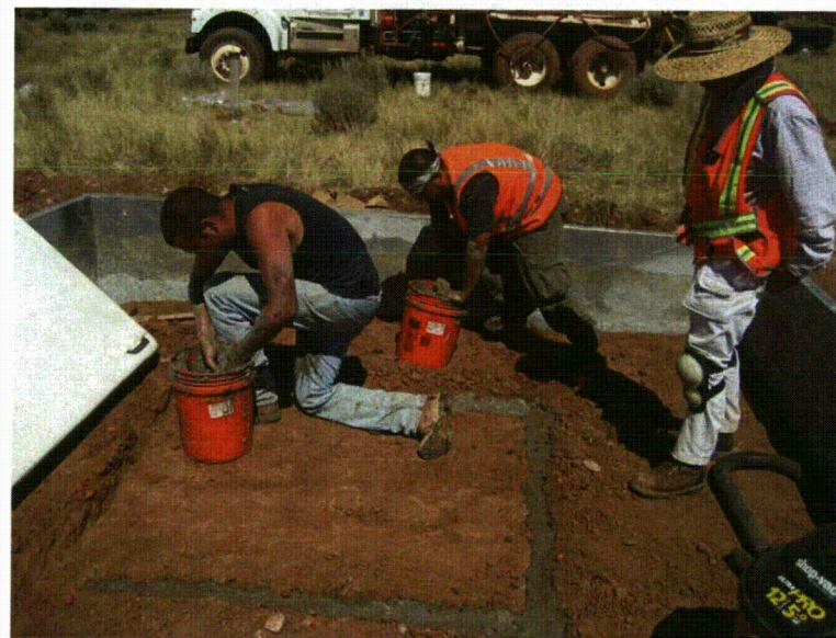
Fig. A.87. Installing bentonite grout for inner TSB ring.
