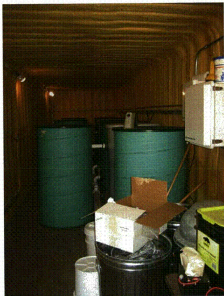
Fig. A.64. Interior of lysimeters and instrumentation trailer.
