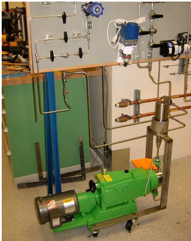
Figure 3-3 System #1 Water Board Shown During Initial Assembly
