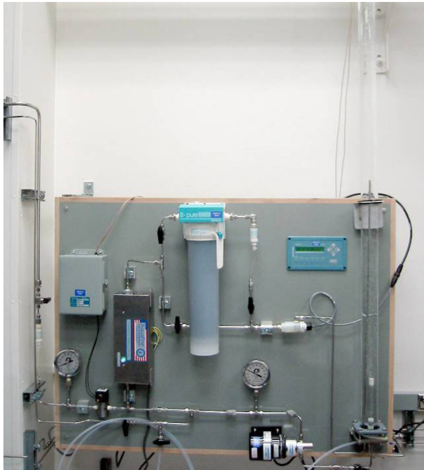
Figure 3-2 Water Make-Up Board is Shown that Produces Ultra-High-Purity Water at a Resistance of 18.18 M ohm-cm. Major components include a UV light box to kill organics, a demineralizer to catch ionic solutes, a submicron filter to catch small inert particles, and a conductivity sensor to measure resistance of the water.
