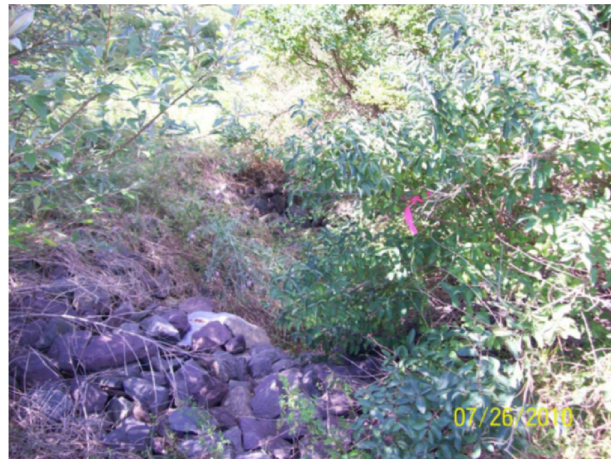
Photo 103. Wetland 49B – culvert outlet to 49C
