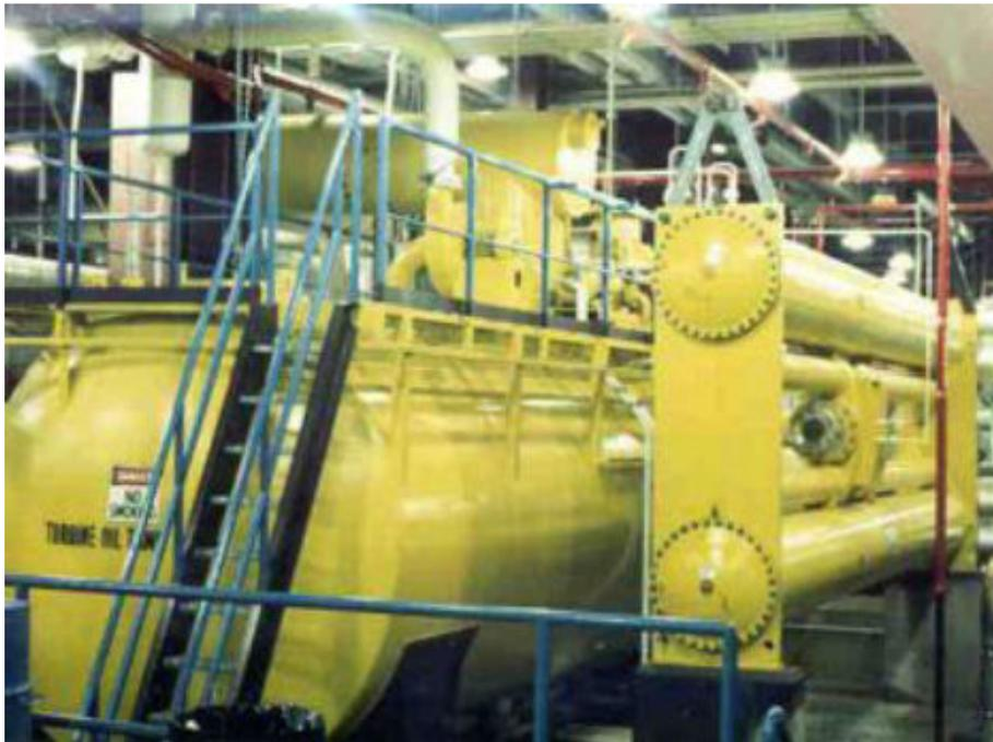
**Figure F-3. The lube oil tank below the turbine deck.**
