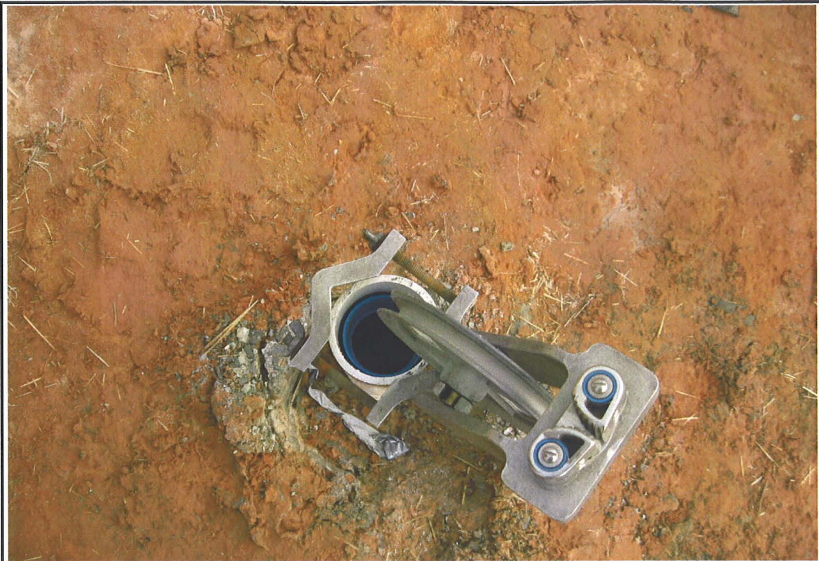
Photo 21. January 22, 2008 – Cross-Hole casing (3" ID, schedule 40, flush coupled PVC) with blue slope indicator casing inside ready to perform the borehole location deviation survey.
