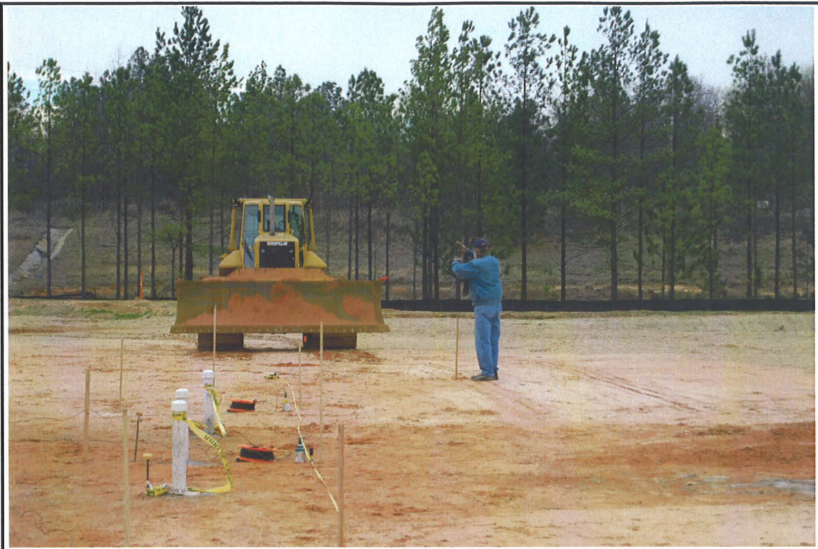
Photo 23. January 24, 2008 – SASW Testing continues with vibrations generated by a bulldozer.
