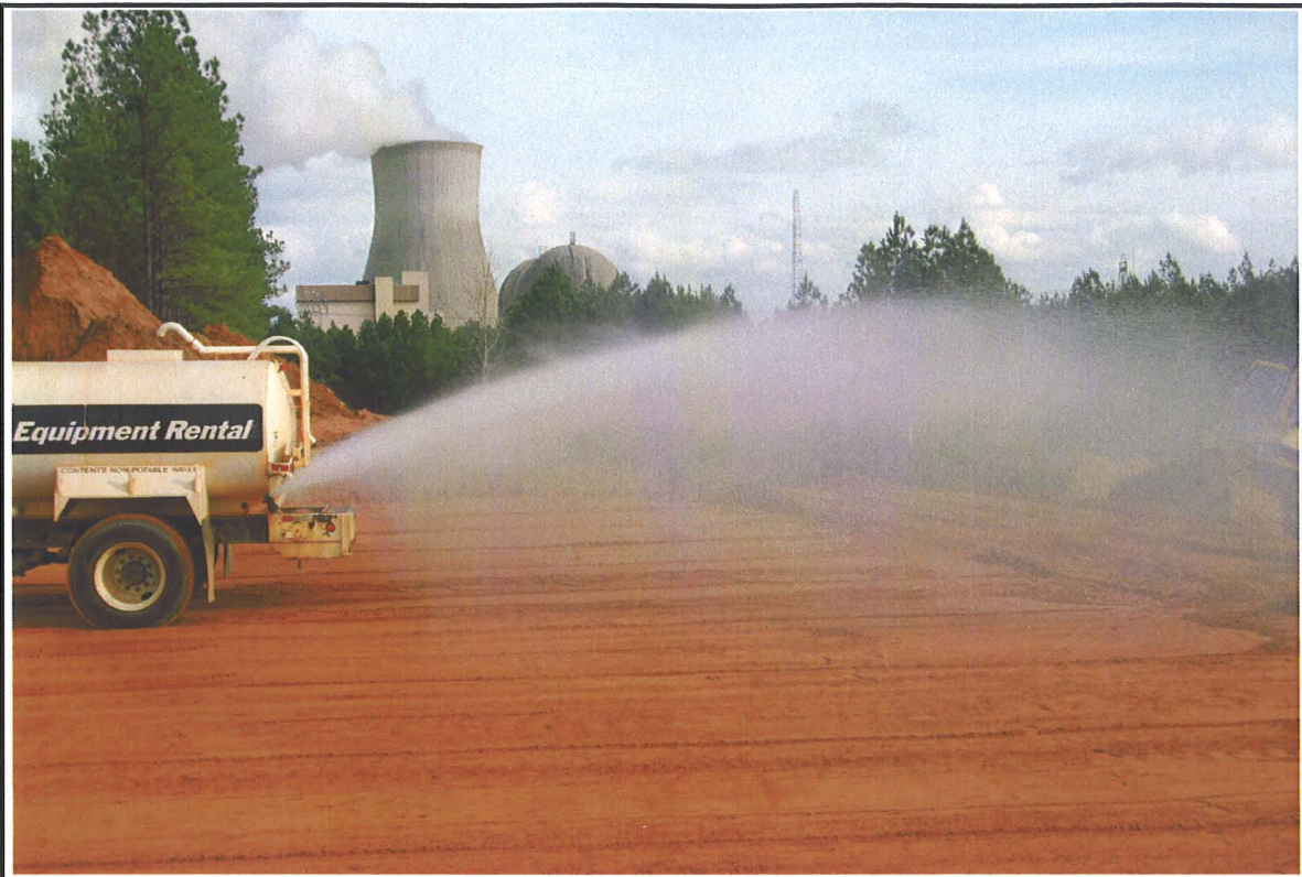
Photo 17. January 10, 2008 – Moisture conditioning of fill lift prior to compaction.
