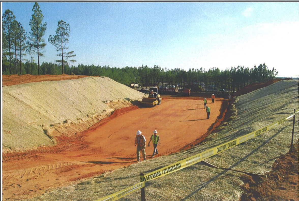
Photo 14. December 10, 2007 – Vibratory compaction of test pad fill continues.
