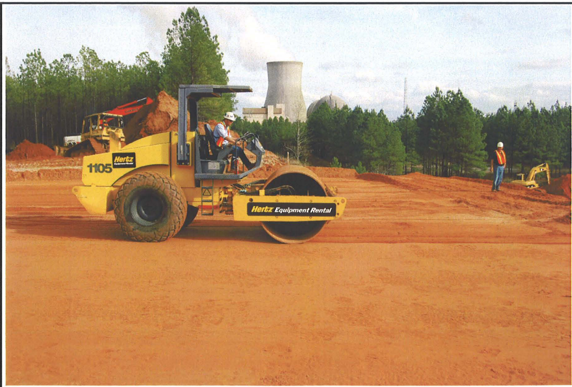
Photo 18. January 10, 2008 – compaction of fill lift with Vibromax 1105 vibratory roller.
