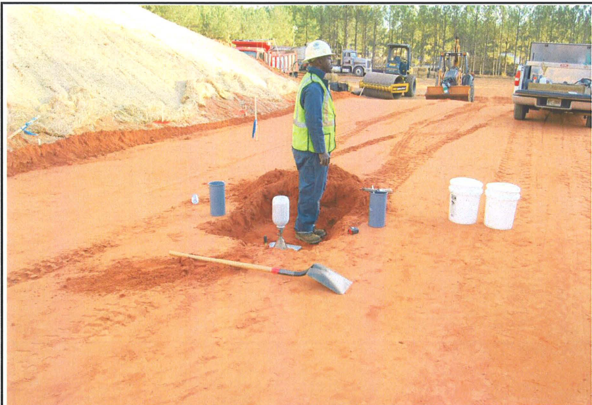
Photo 8. December 4, 2007 – Sand cone density test is underway by Roger Blalock. Two 5-gallon bulk samples will be obtained from the density test layer for testing.
