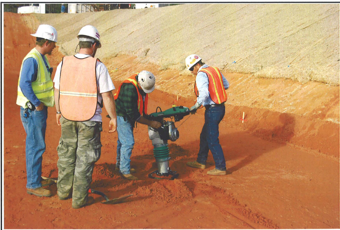
Photo 10. December 5, 2007 – A sand cone density test excavation is being repaired with a “Wacker Packer”.
