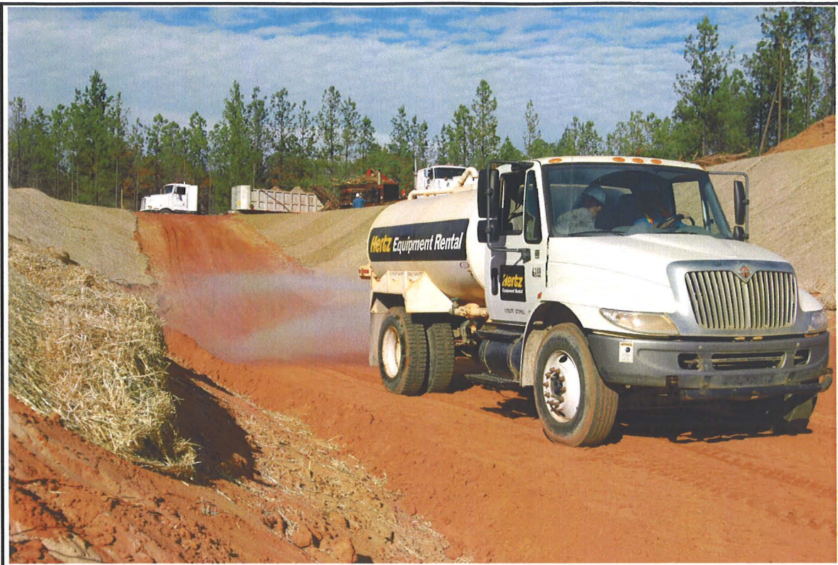
Photo 9. December 5, 2007- Moisture conditioning of fill layer.
