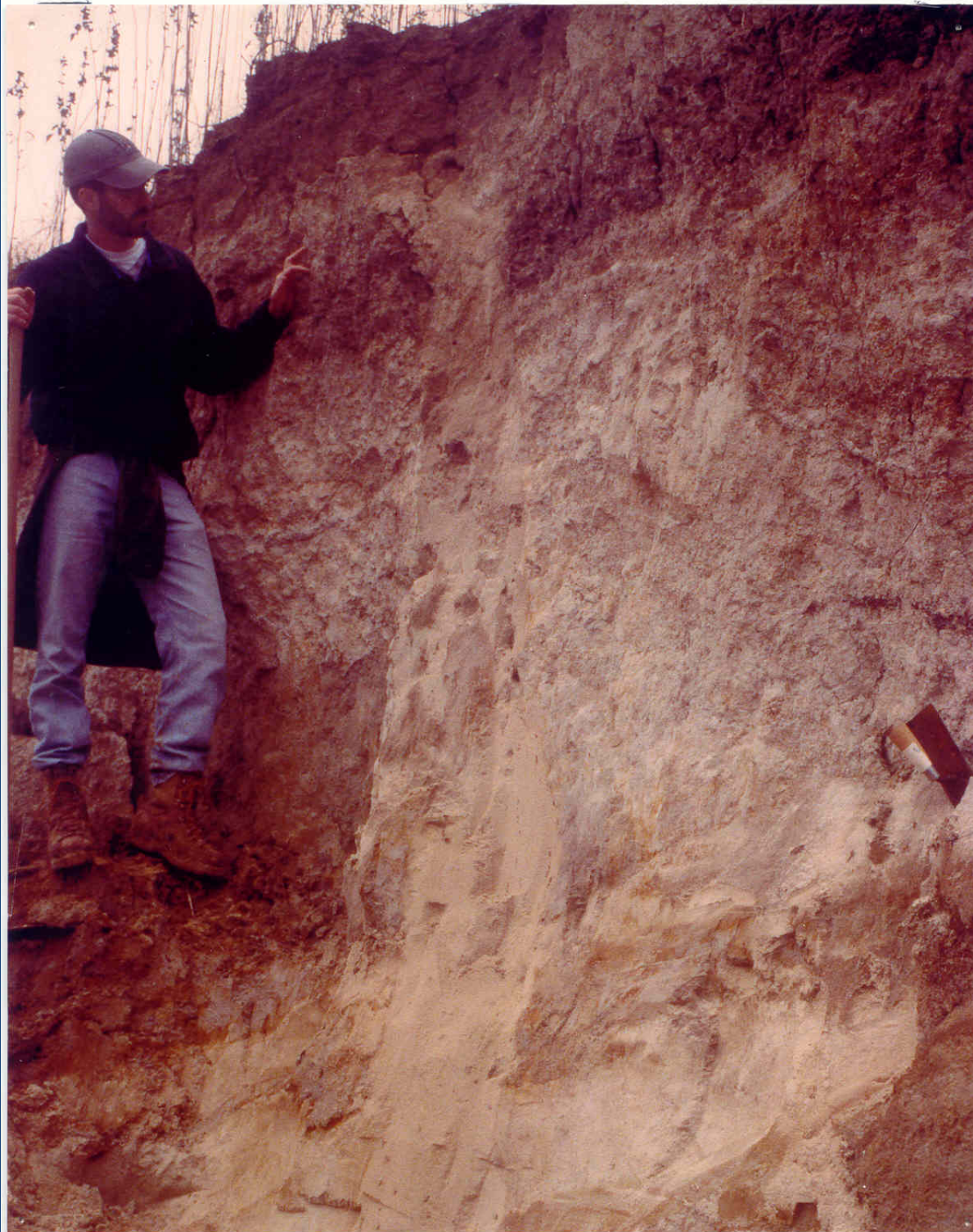
Sand dike in bank of Wolf River in Memphis formed during earthquake liquefaction (from Broughton et al., 2001).
