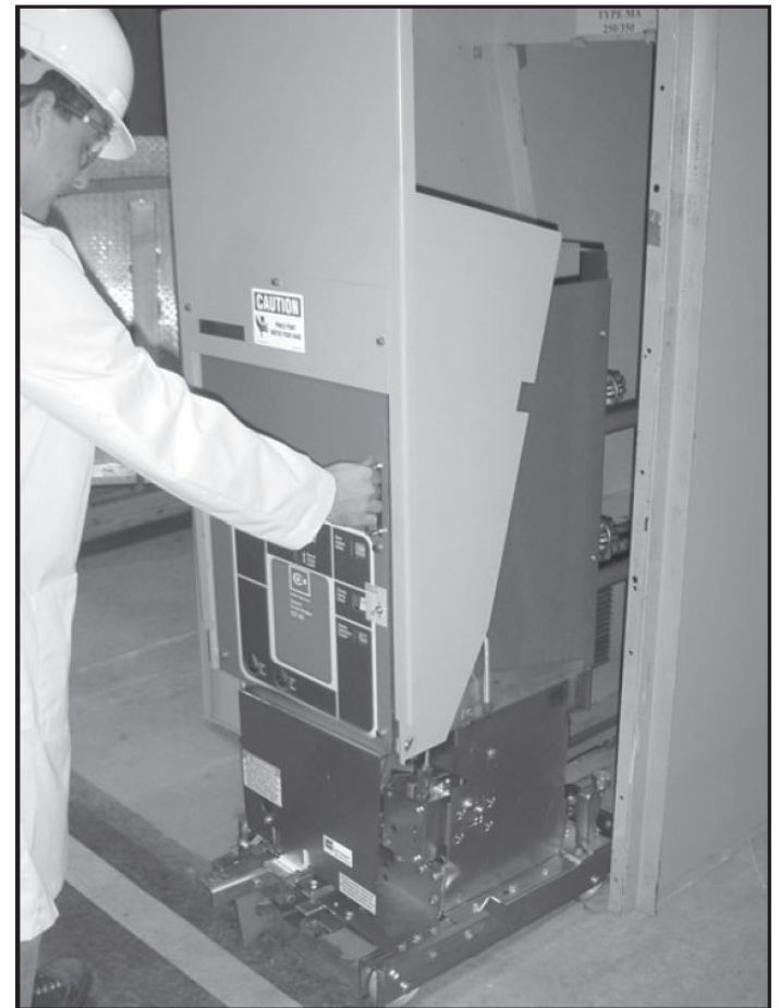
Figure 4-4 Insertion of MA-VR
