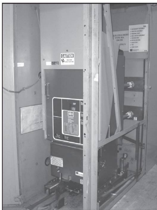
Figure 4-11 Disconnect Position ①
