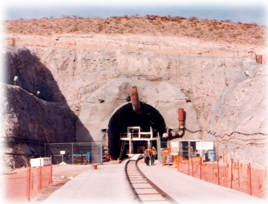
Entrance Tunnel at Yucca Mountain
