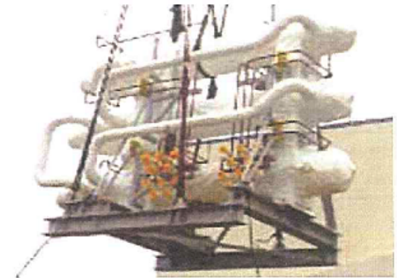
CUW Heat Exchanger Module
