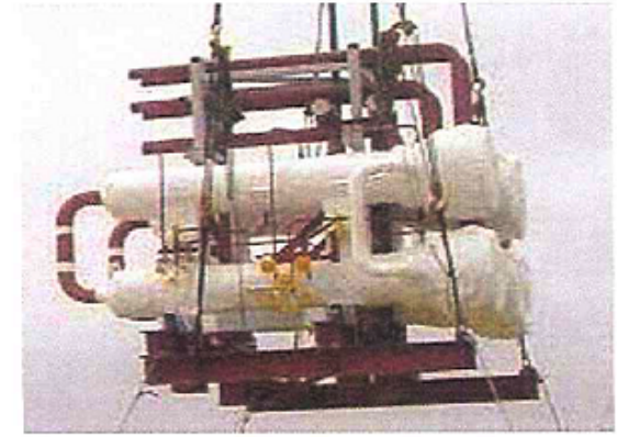
CUW Reheat Exchanger Module
