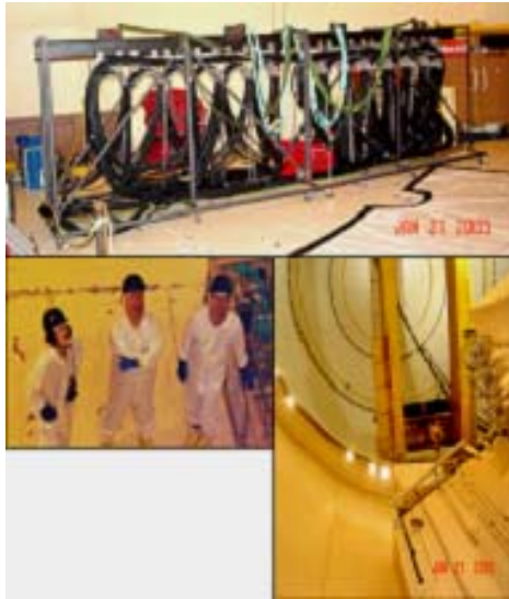
Polar Crane Modifications
