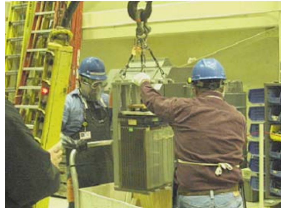
Lifting battery cells
